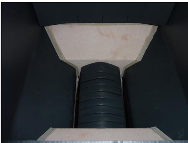
CxxS, ACxxS, KCxxS boiler gasifier grille without special additional grille
