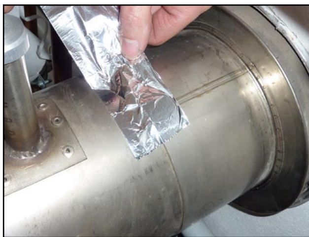
Tightening the flue with an aluminium tape
