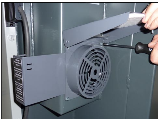
Assembling valve under flap with grille
