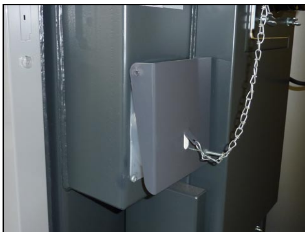
Closed flap for inflow of combustion air for DCxxSP boiler
