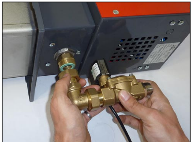
Take complete screw fitting with solenoid control and connecting cable and screw it to the burner
