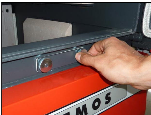
Tightened additional secondary air cap for DxxP boiler
