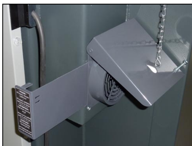
Open valve and regulating flap when burning with manually added fuel
