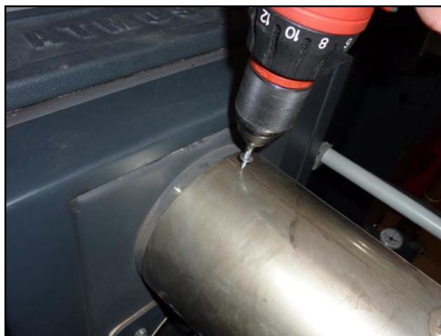
Securing the flue with a screw
